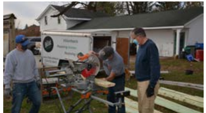
The Build Team at work. Photo by Tom Benjamin.
