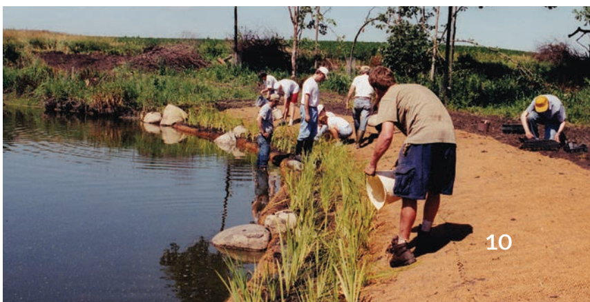
FLINT CREEK STREAM BANK STABILIZATION - CFC PHOTO ARCHIVE
